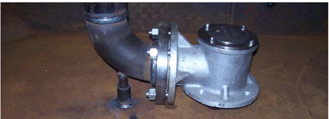
Inside view of a Transtank showing Anti-syphon Valve
