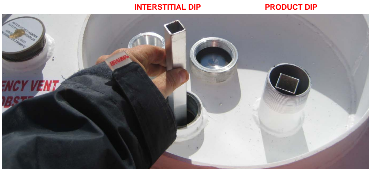
Top view of Transtank showing Dip Sticks
